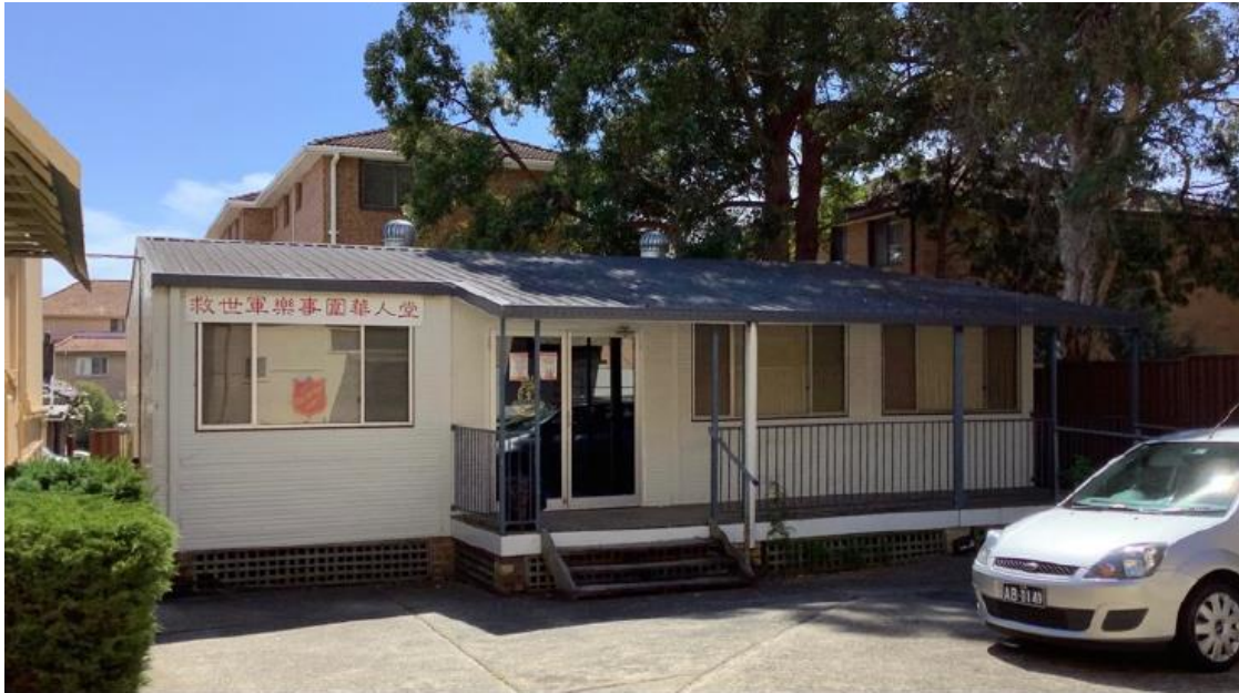
Figure 6 Demountable building at the rear of 22 Bond Street
