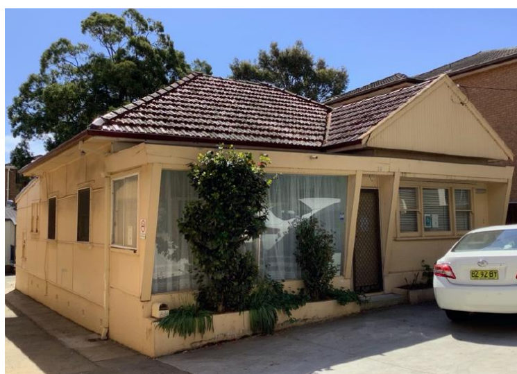
Figure 5 Vacant House at 22 Bond Street
