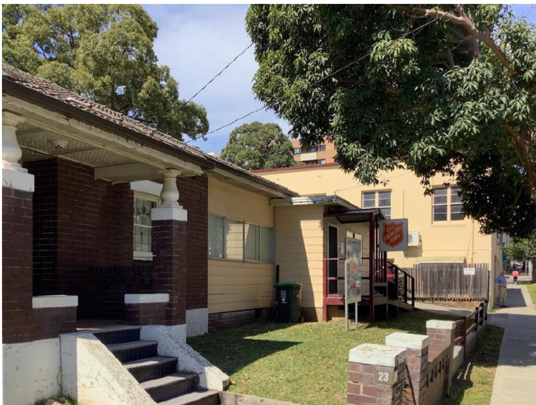
Figure 7 The Admin and Money Care Building from Dora Street
